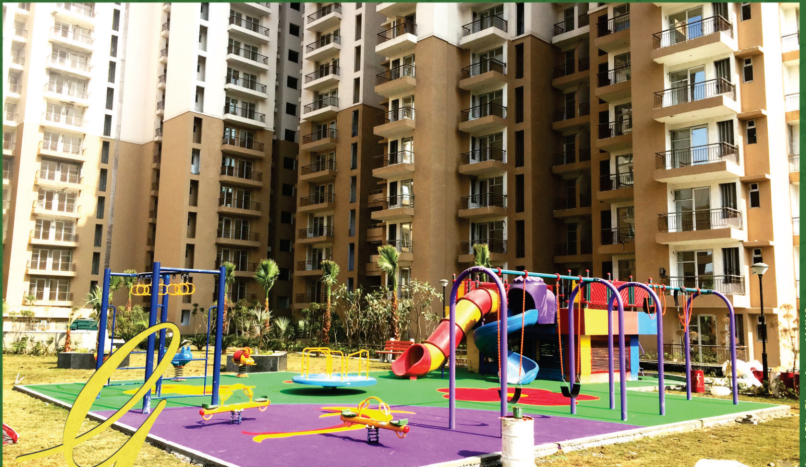
Actual Site Photo As on JAN'18
